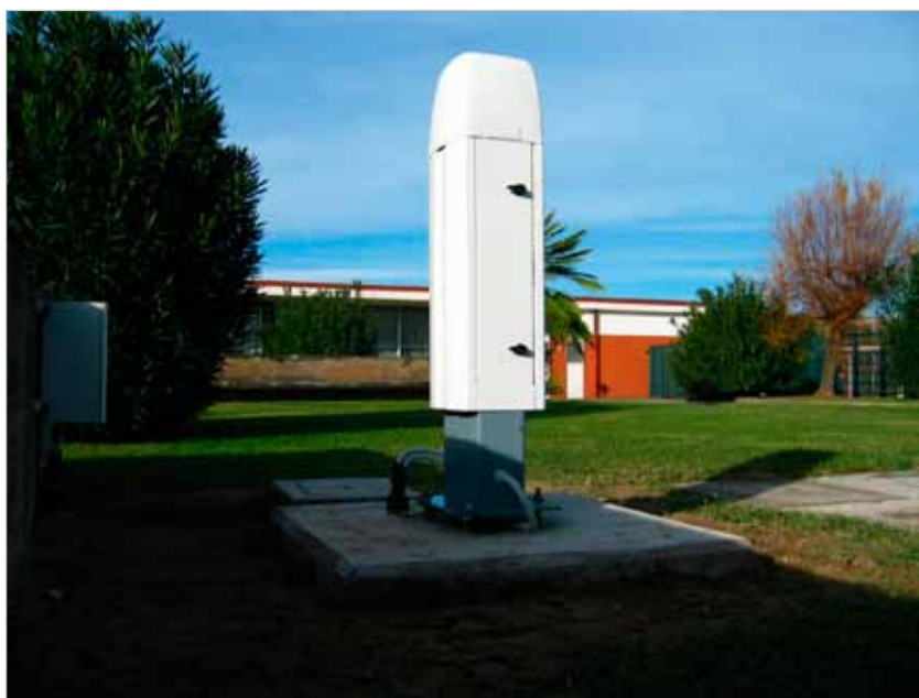
CL31 Ceilometer installed at COSIB in Termoli, Italy.
